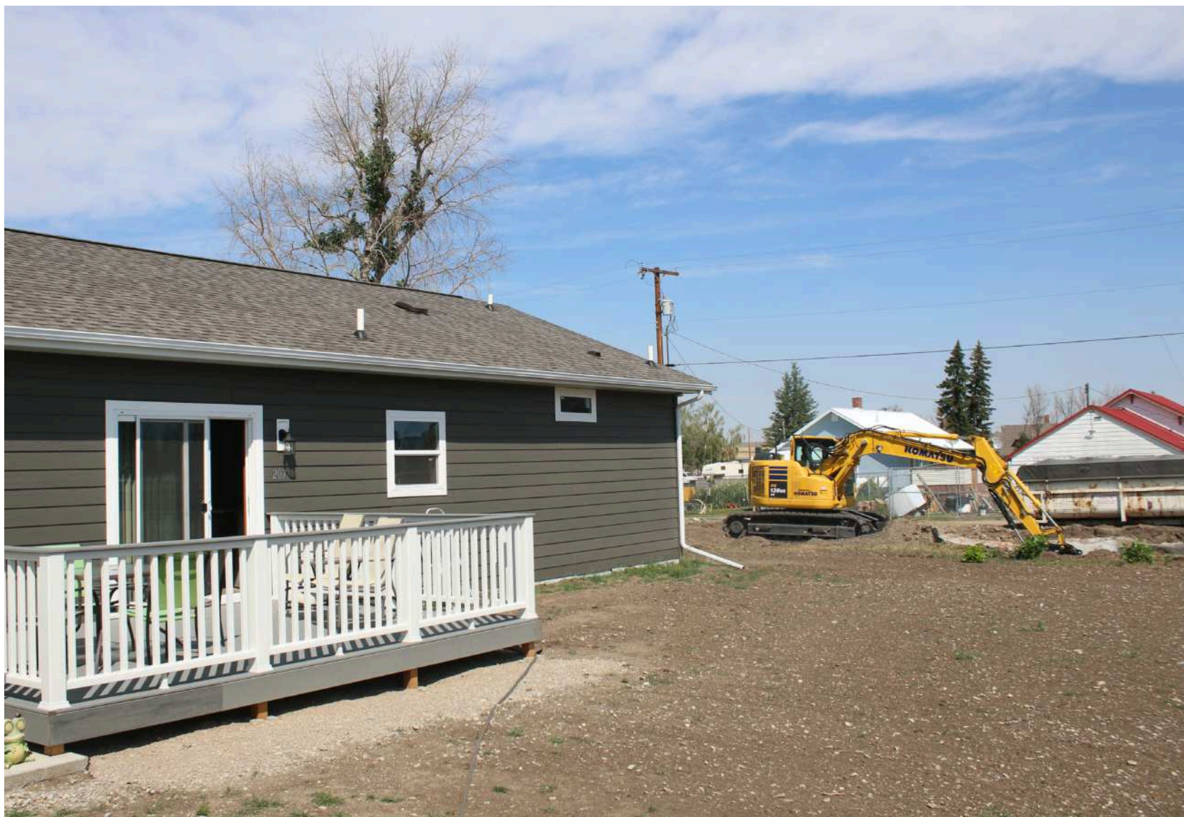
While Erlandson’s house is the first new home built in Denton since the West Wind Fire in December, many of her neighbors are still recovering. The lot next door to hers, as pictured here, is the last in town to be cleared. Photo by Will Briggs
