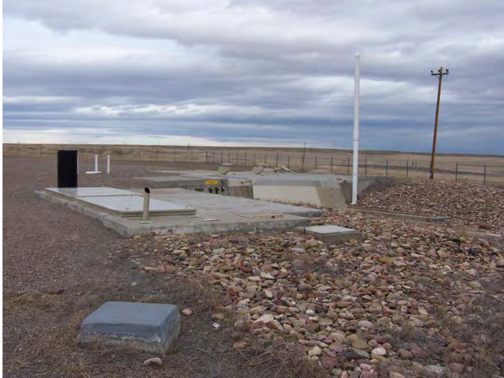
Photograph A-3. LF J-10 Surface view.
