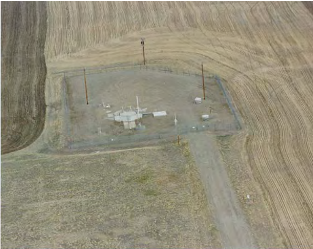
Photograph A-2. LF T-44 Aerial view.
